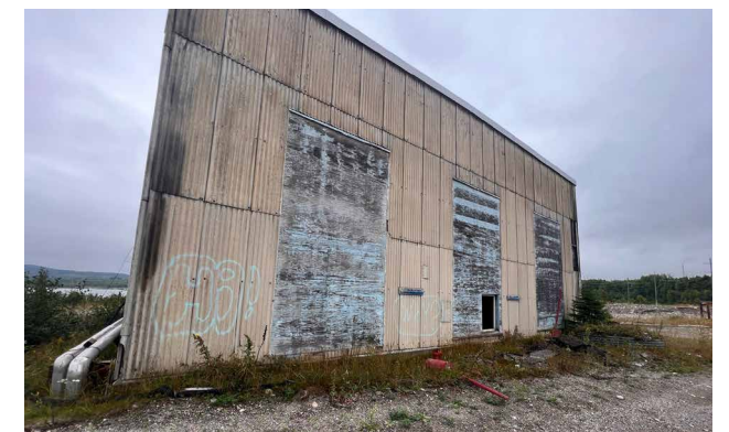
The only industrial building left
