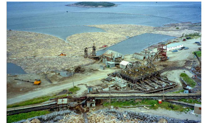
Boom and Jack ladder, 1983/84
